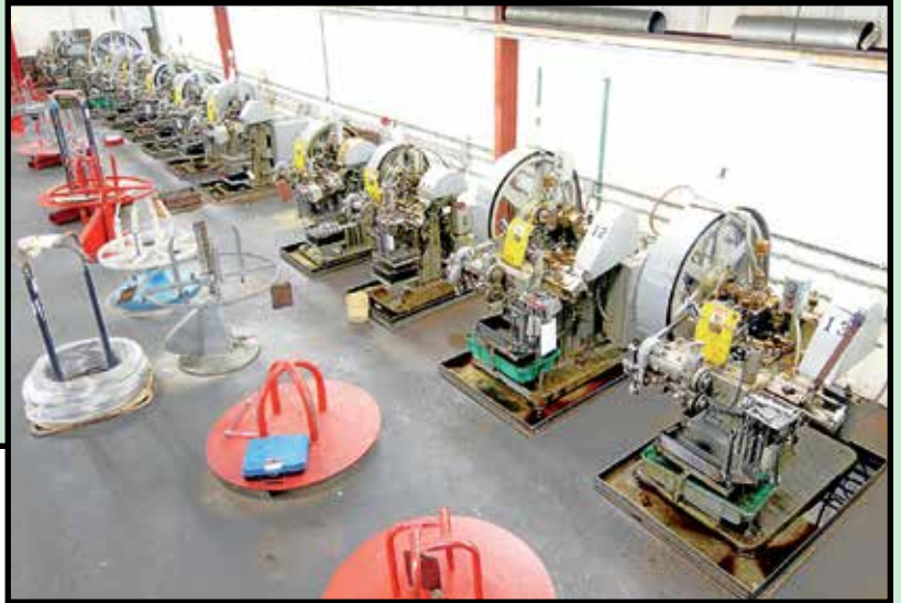
VIEW OF WATERBURY HEADERS
