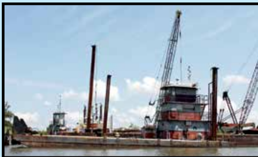
< M/V POKO SELF-PROPELLED WORK BARGE
