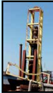
PNEUMATIC PILE DRIVER
