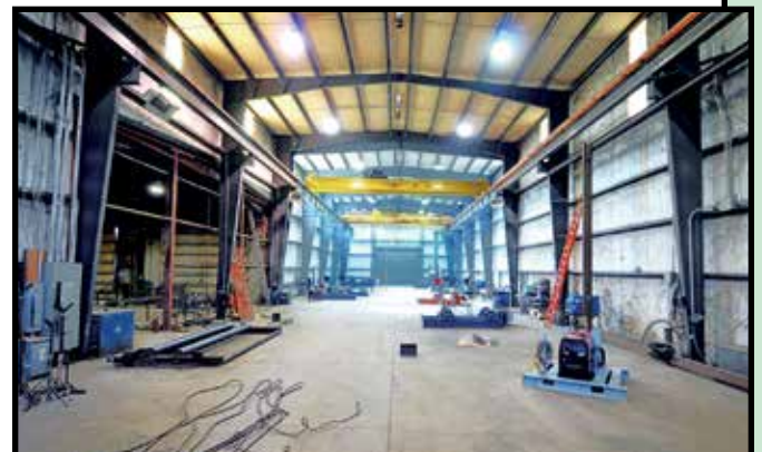
INTERIOR VIEW OF MAIN FABRICATION BAY
