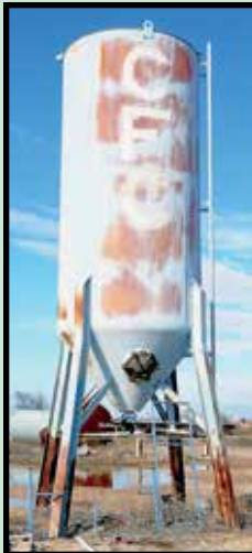
SAND BLAST TOWER
