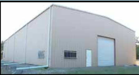
(1 OF 6) BUILDINGS ON THE PROPERTY
