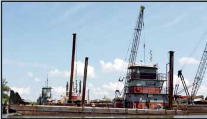
M/V POKO SELF-PROPELLED WORK BARGE
