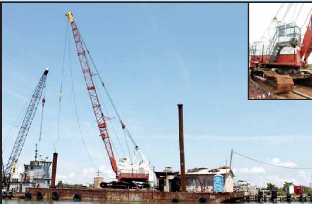
NORTHWEST CRANE AND KS 393 SPUD BARGE
