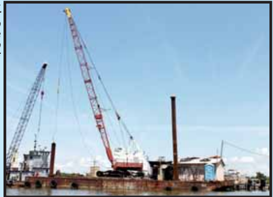
> NORTHWEST CRANE AND KS 393 SPUD BARGE
